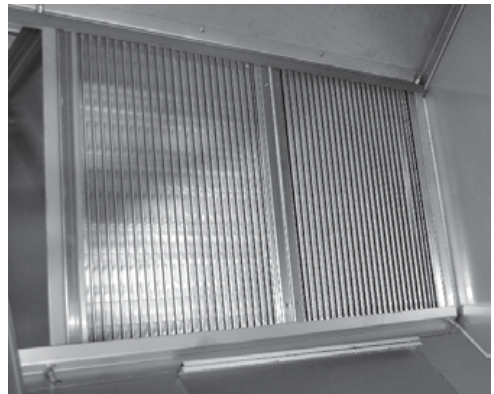
Plate recuperator (Fig. 25)
