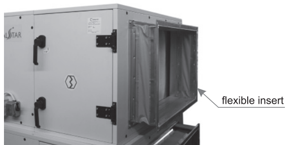
Connecting air ducts (fig. 10)
