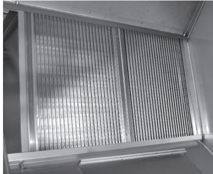
Plate recuperator (Fig. 12)
